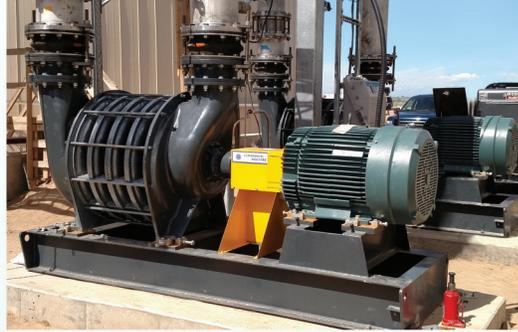
*Two (2) Model 151.05 packages with 125 HP motors at Methane Waste to Energy facility in Colorado.*
